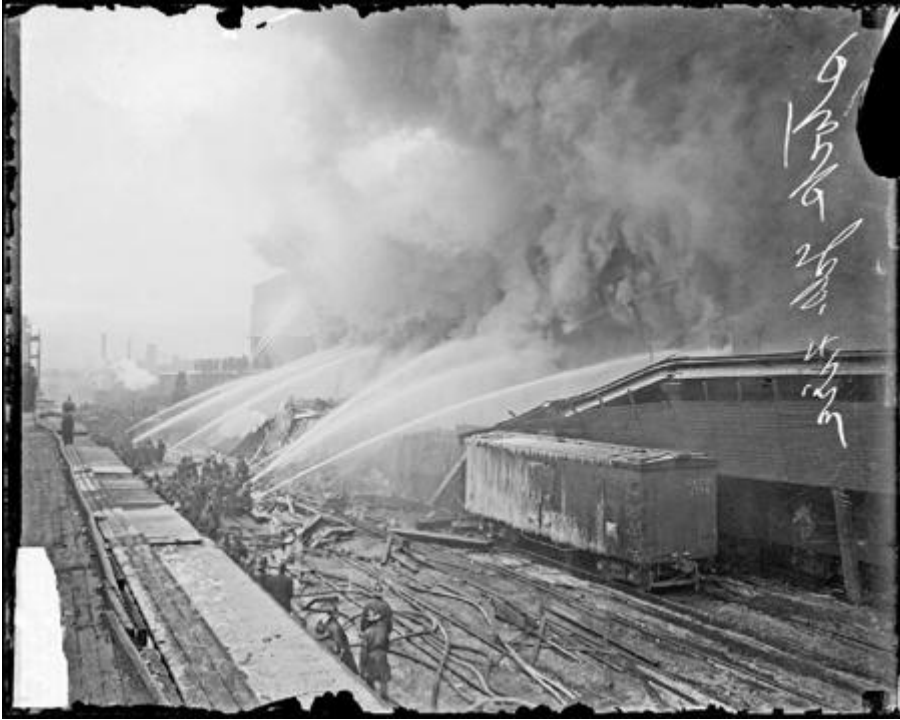
A row of railcars separated the firemen from the burning building, hindering firefighting efforts. Photograph by the Chicago Daily News
