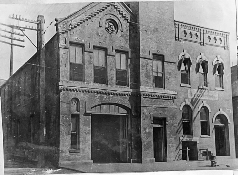
Former house of ENGINE 29 and the Deering police district station located at 744 W. 35 TH Street in the section of Deering, that was razed in 1920. ENG 29 remained here in an old horse barn on the back lot until new house was finished at 3509 S. Lowe Avenue, and occupied it on May 19, 1925. ( John McIntre collection )
