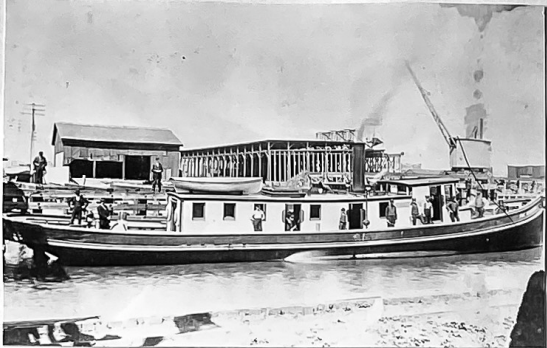
CHICAGO (E58) ORIG 95th St. BRIDGE HIST SOC 1894
