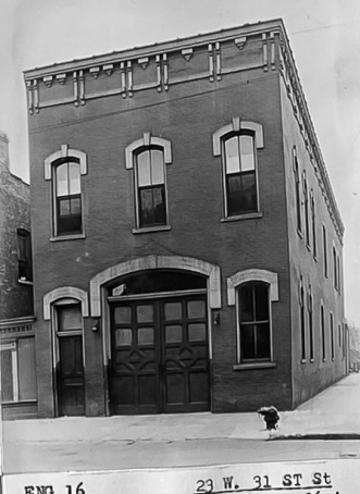
ENG 16 23 W. 31 ST St Put in service here in the 1860's this old structure was occupied by company until Oct 24, 1960 and company moved to ENG 48, Batt 10 to new house of ENG 19 and TRK 11.
