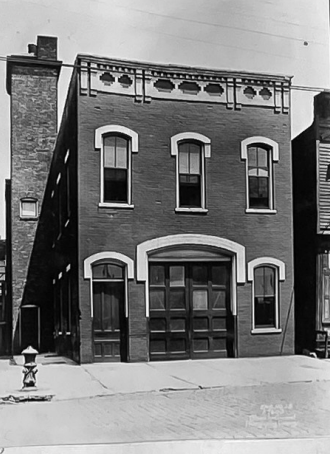
ENG 15 1156 W. 22 ND St Organized here in this building ENG 15 remained until disbandment on Feb 2, 1932 to be re-organized at 8028 S. Kedzie Ave in Scotsdale on Apr 4, 1957 with Truck 59.
