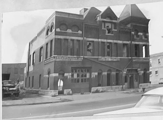
House of Truck 18 comes down under weight of wreckers hammer at Halsted & 48 TH; it was formally the town hall of the City of Lake years ago before Lake was annexed to CHICAGO. Circa 1961 (CV)
